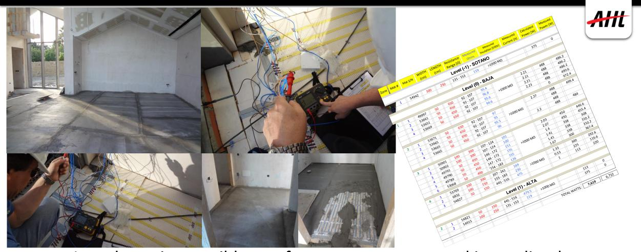
In order to insure ribbon safety, cement was casted immediately after mats were put into place, not before each mat was tested and recorded for resistance, current and insulation resistance!!
